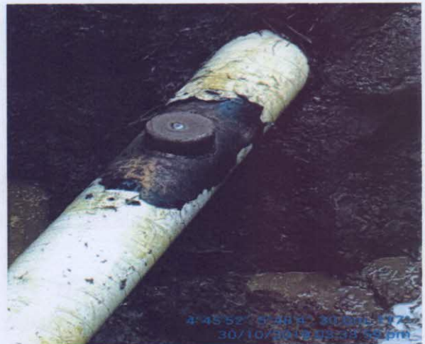
Fig F: Incident point after repairs
